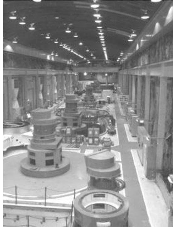
Soon after the power station commenced full operation in 1972 engineers discovered a design problem. The friction between the water and the walls of the tailrace tunnel effectively resulted in a reduced hydrodynamic head. Until the second tunnel was constructed in 2002 the operators risked flooding the powerhouse if they ran the station at an output greater than 585 MW. This was far short of the planned output of 700 MW.
