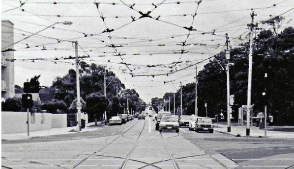
Such a junction on a tramway is quite rare being a crossroad with four junctions, one to each street. Apart from the interesting rails, just take a look at the overhead system required to achieve this. What a headache for the designer, not least to the linesman erecting it all. The tram picture portrays a Class B tram on route 96 to St. Kilda.
